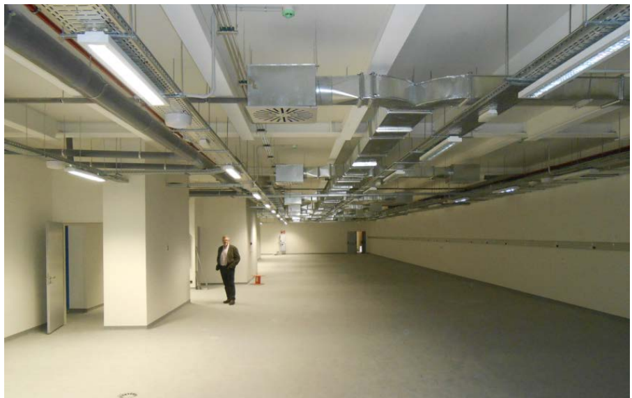
Laboratory area of the ground floor of M5, as in May 2013. It is empty but with a predesign to panel it in a flexible way
