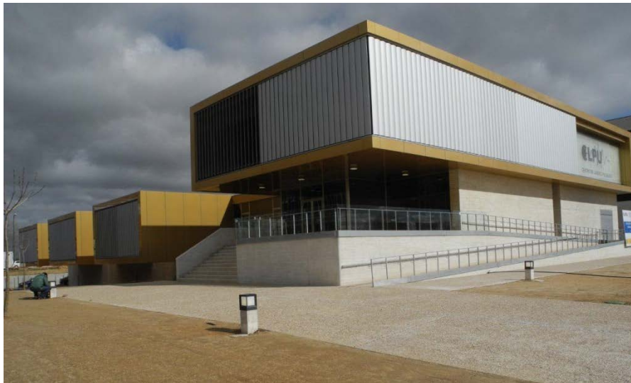
Headquarters of CLPU, the M5 building
